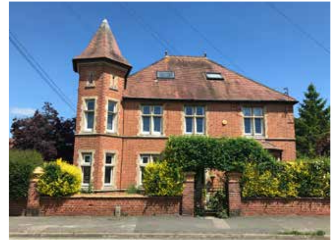
Figure 09: Example of grand Victorian manor house, with typical red brick finish and stone window casing
