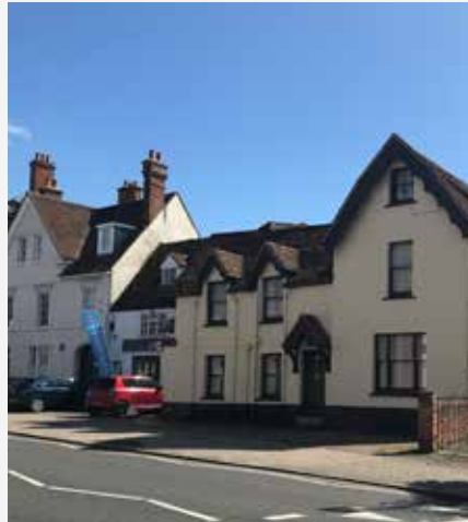
Figure 41: Front facing gables, High St
