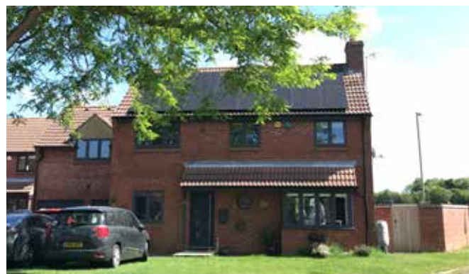
Figure 169: Solar panels on existing home, Howlands Road
