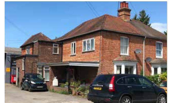
Figure 157: Unsympathetic side extension
