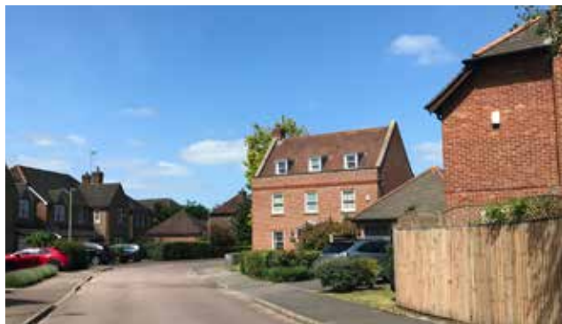
Figure 159: Outbuilding with hipped roof and in consistent, contextually sensitive materials
