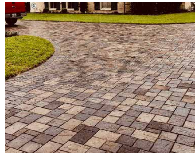
Figure 177: A good example of permeable paver (Source: https://www.paverconnection.com/testimonial/hedwig-village-permeable-driveway-and-patio-upgrade/ )
