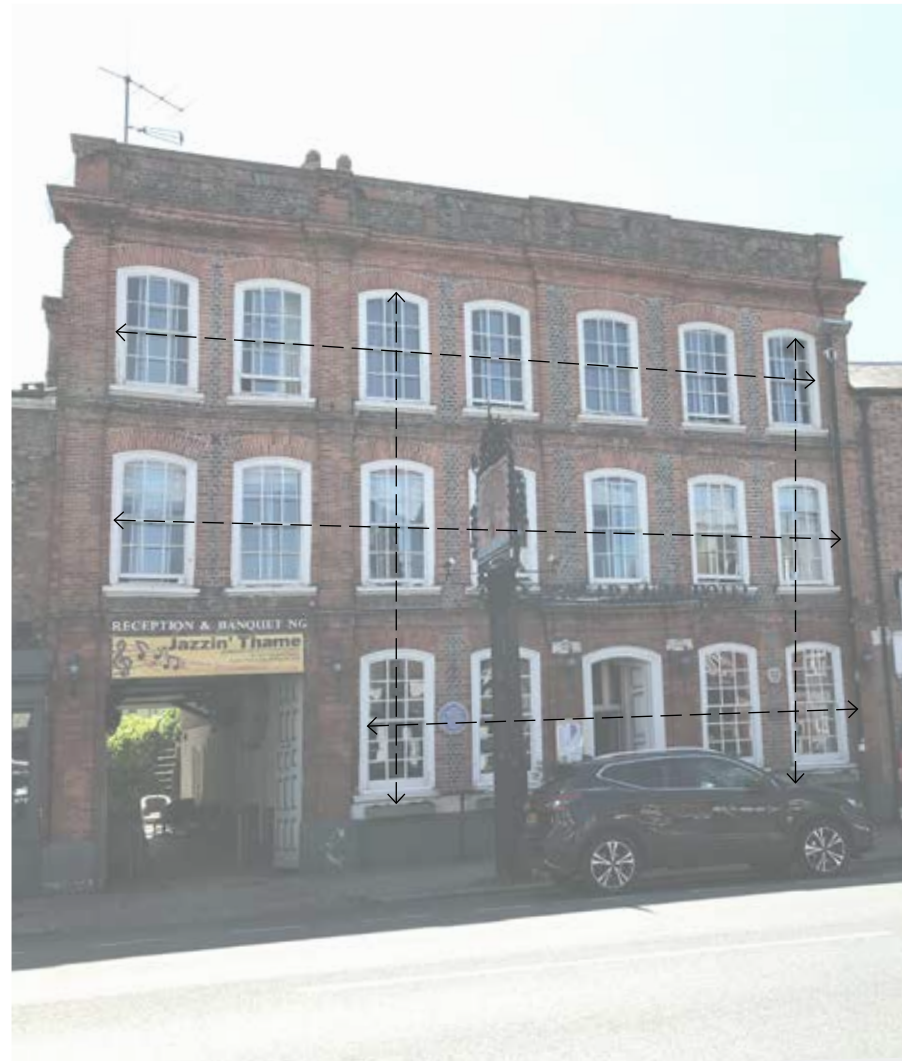
Figure 132: Repeated rhythm on Georgian facade creates regular proportions
