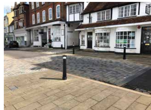
Figure 88: An example of raised pedestrian crossing with a plateau in Hemel Hempstead
