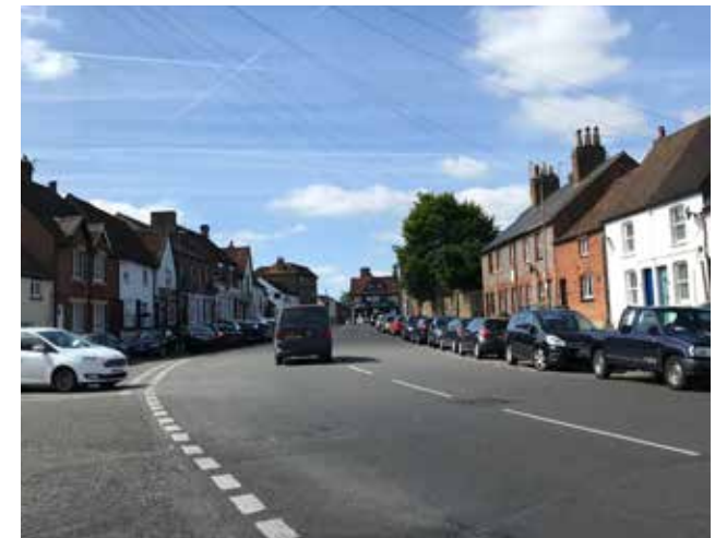
Figure 138: 1:4-6 enclosure along North Street
