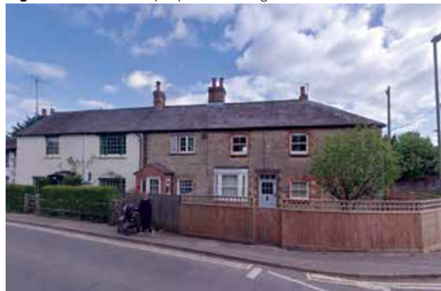
Figure 114: Buildings of note along North Street
