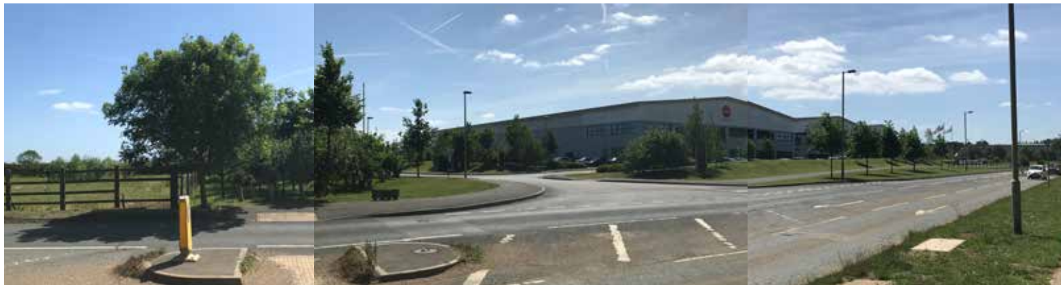
Figure 166: View south along B4012, at the entrance point to Windles Group
