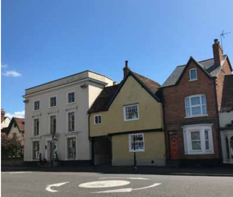
Figure 32: Northern end of High Street
