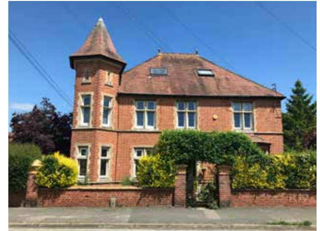
Figure 05: Example of grand Victorian manor house, with typical red brick finish and stone window casing
