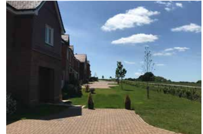
Figure 60: View west from Causeway Close
