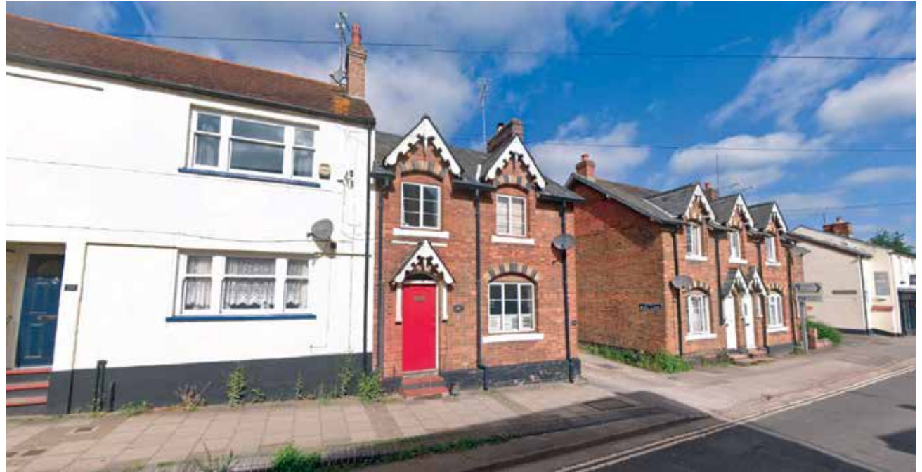
Figure 113: Victorian properties along North Street
