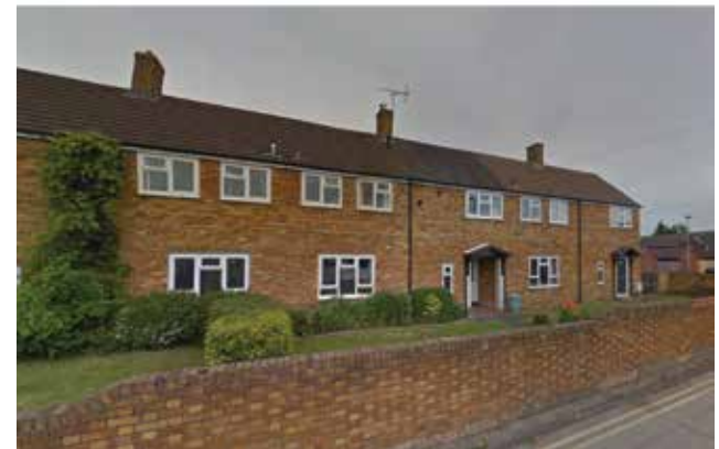
Figure 115: View east along Abingdon Close
