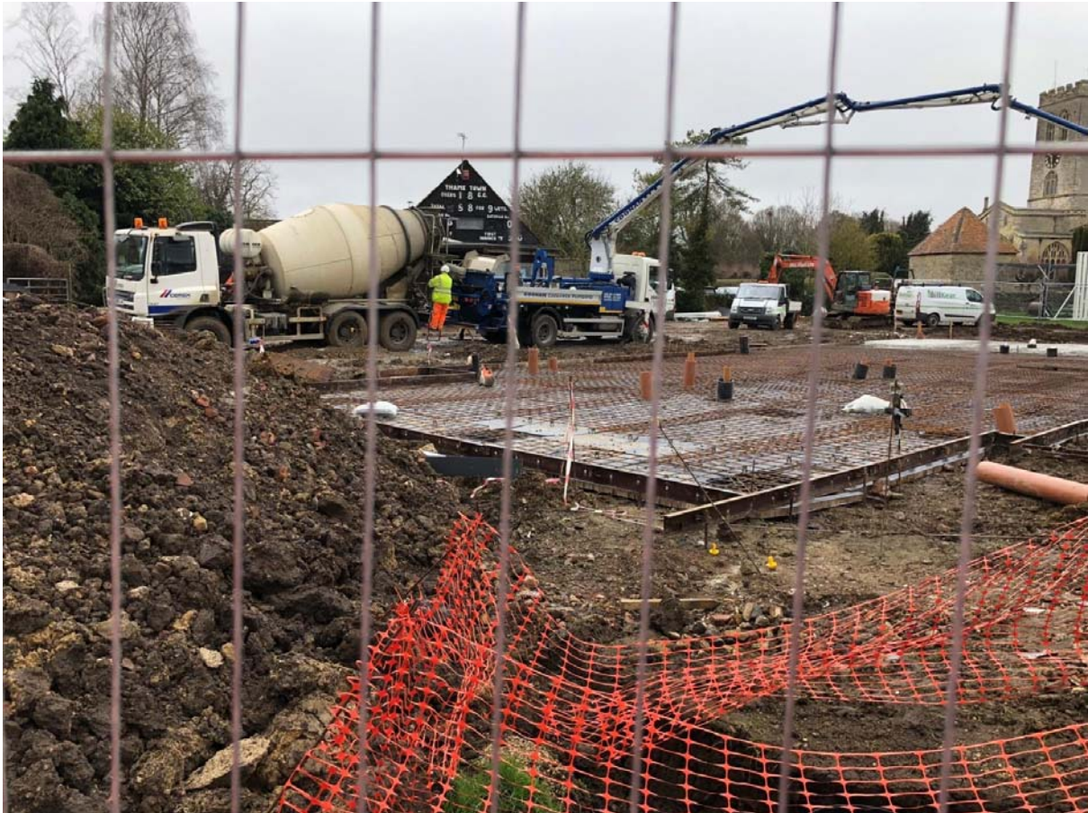
Concrete slab being poured
