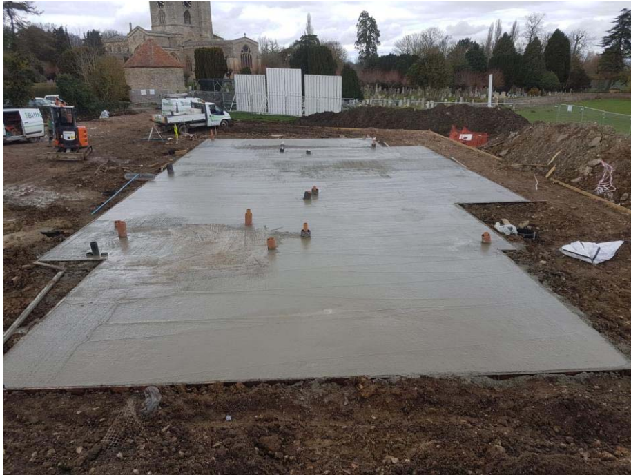
Concrete slab completed
