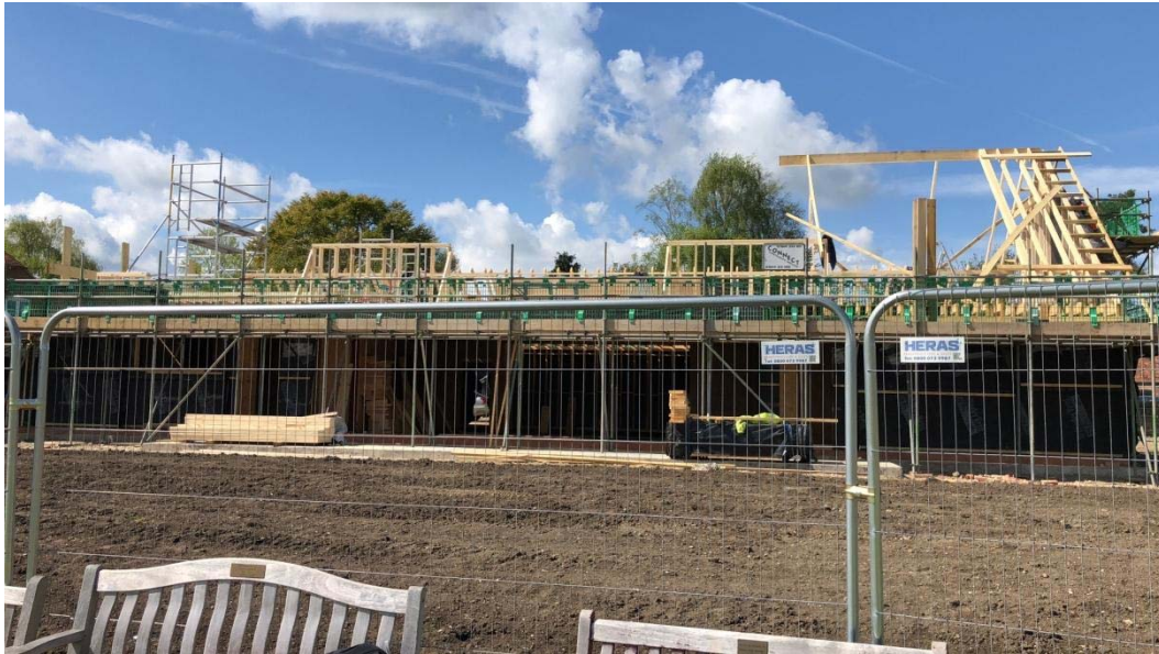
Roof works continue with scaffolding in place
